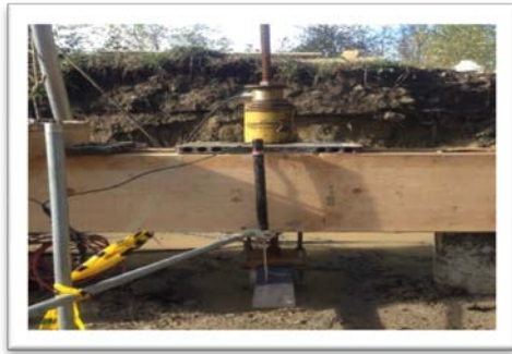
Figure 3. Pile load test in the Gloucester site
