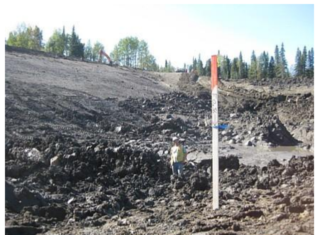
Figure 5. Subgrade preparation in wet conditions.
