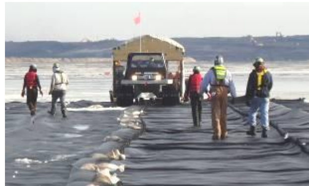
Figure 4. Placement of geotextile on frozen tailings pond.
