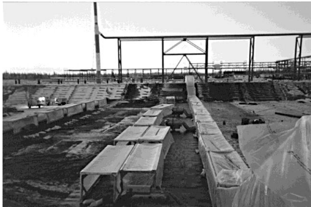
Figure 3. HDPE installation using temporary shelters.
