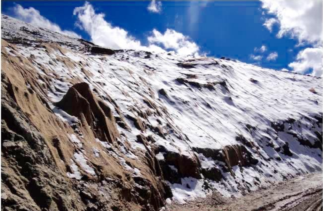
Figure 6. Stabilized hill slope with jute geotextile (JGT).
