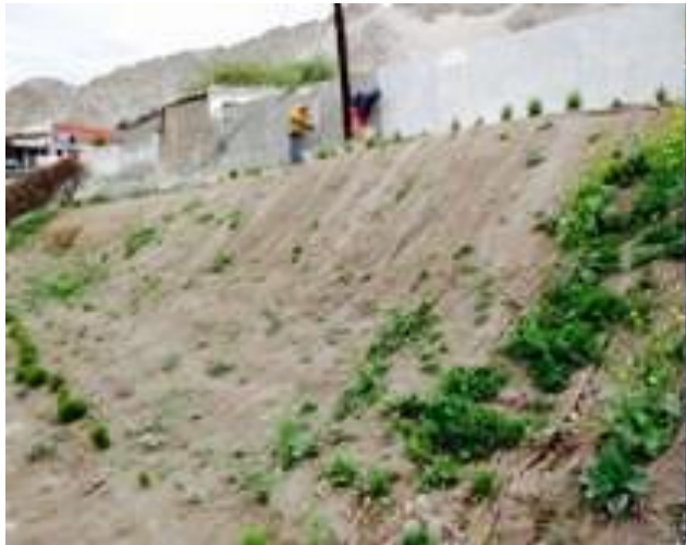
Figure 5. Application of jute geotextile (JGT) and its vegetative growth effect.
