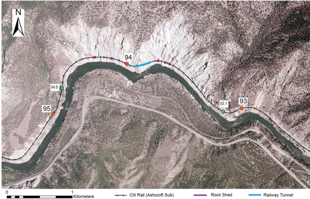
Figure 5: The White Canyon corridor extends from Mile 93.1 to Mile 94.6 on CN's Ashcroft sub. The location of the tunnel dividing the West and East portions of the slope, as well as the six rock sheds is shown.
